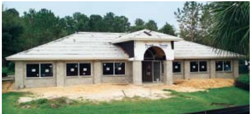
Constructing Vernon Center!
